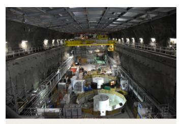
A July 2018 view from the service tunnel into the powerhouse cavern. Two of the three turbines/generators are the circular works.
